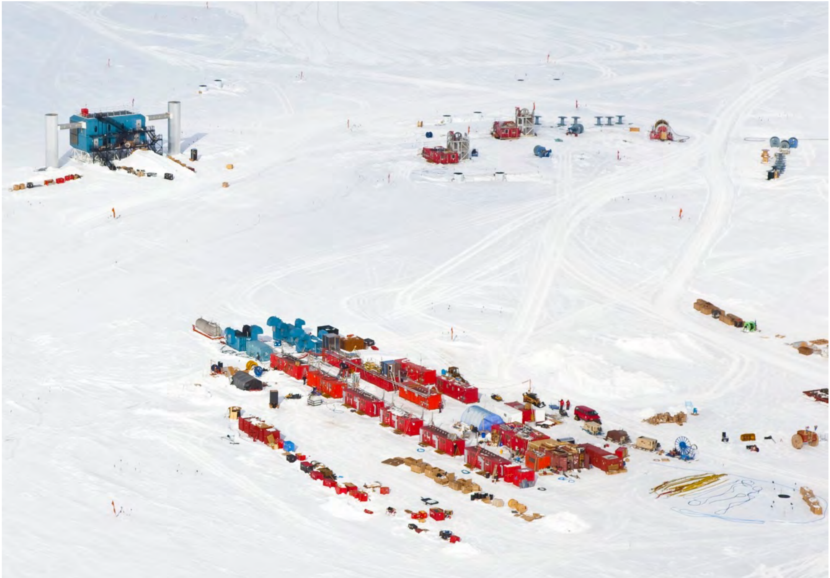
IceCube construction 20 Seasonal drill camp
