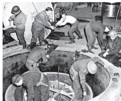
Fig. 10. Equipment ‘Haigerloch pile being dismantled as part of the Alsos mission, Haigerloch, Germany (date unknown). Credit: AIP Emilio Segre Visual Archives, Goudsmit Collection.
