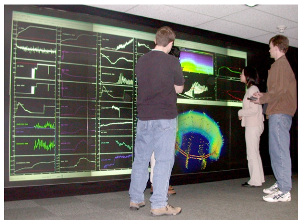
Tiled display walls with shared visualizations and communication are being installed to create collaborative fusion experimental control rooms.
