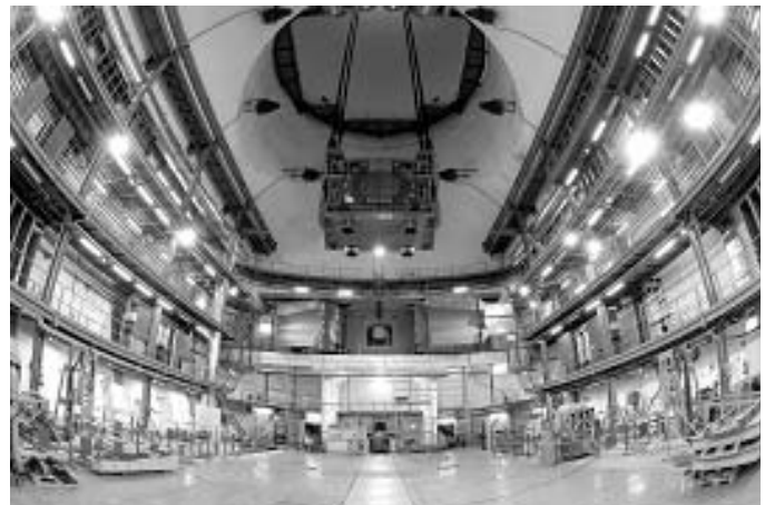
Lowering of CMS Detector Components into the Experimental Cavern
