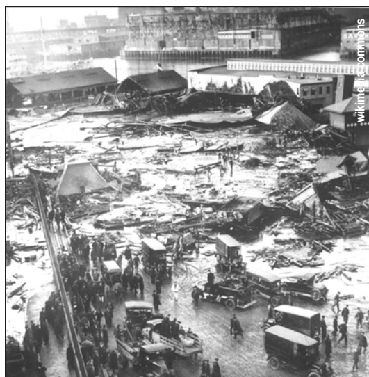
Aftermath of the rupture of a tank of molasses in Boston, January 15, 1919.
